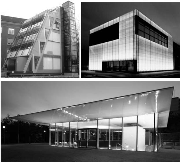
*Fig. 4. Examples of buildings partially or entirely made of FRP. On the top-left the Eyecatcher Building that represents one example of a building made entirely by GFRP. On the top-right is the Regent Lighting Center constructed in Basel with a translucent shell of GFRP panels. On the bottom, the roof of the Main entrance of the Novartis campus in Basel, it is entirely made by light-weight GFRP*
